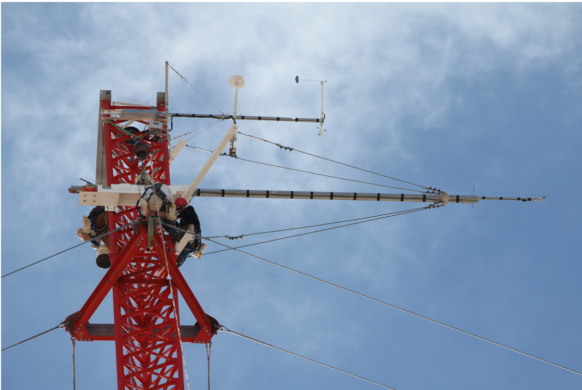
Figure 5. Torque arm at 130 m on the M4 mast. The torque arm is the large, triangular frame connected to guy lines leading out of the photograph. The sonic anemometer boom at 131 m a.g.l. is being installed. The cup anemometer and vane at 134 m a.g.l. are also visible. Photo courtesy Lee-Jay Fingersh, NREL.
