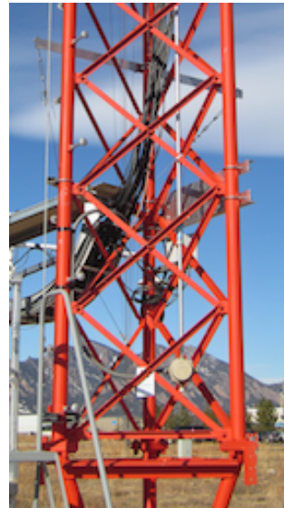
(b) Elevation view of the base of the M5 mast. The 3-m boom is visible above the cable gantry (left). Photo courtesy Lee-Jay Fingersh, NREL
